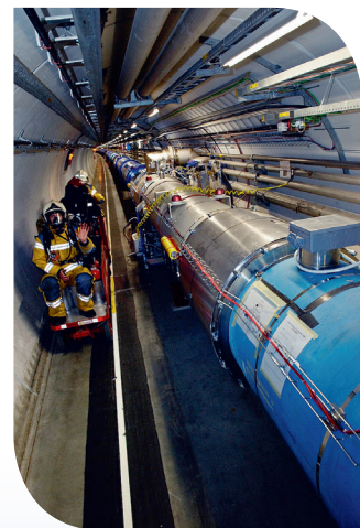
Tunnel LHC, photo CERN
